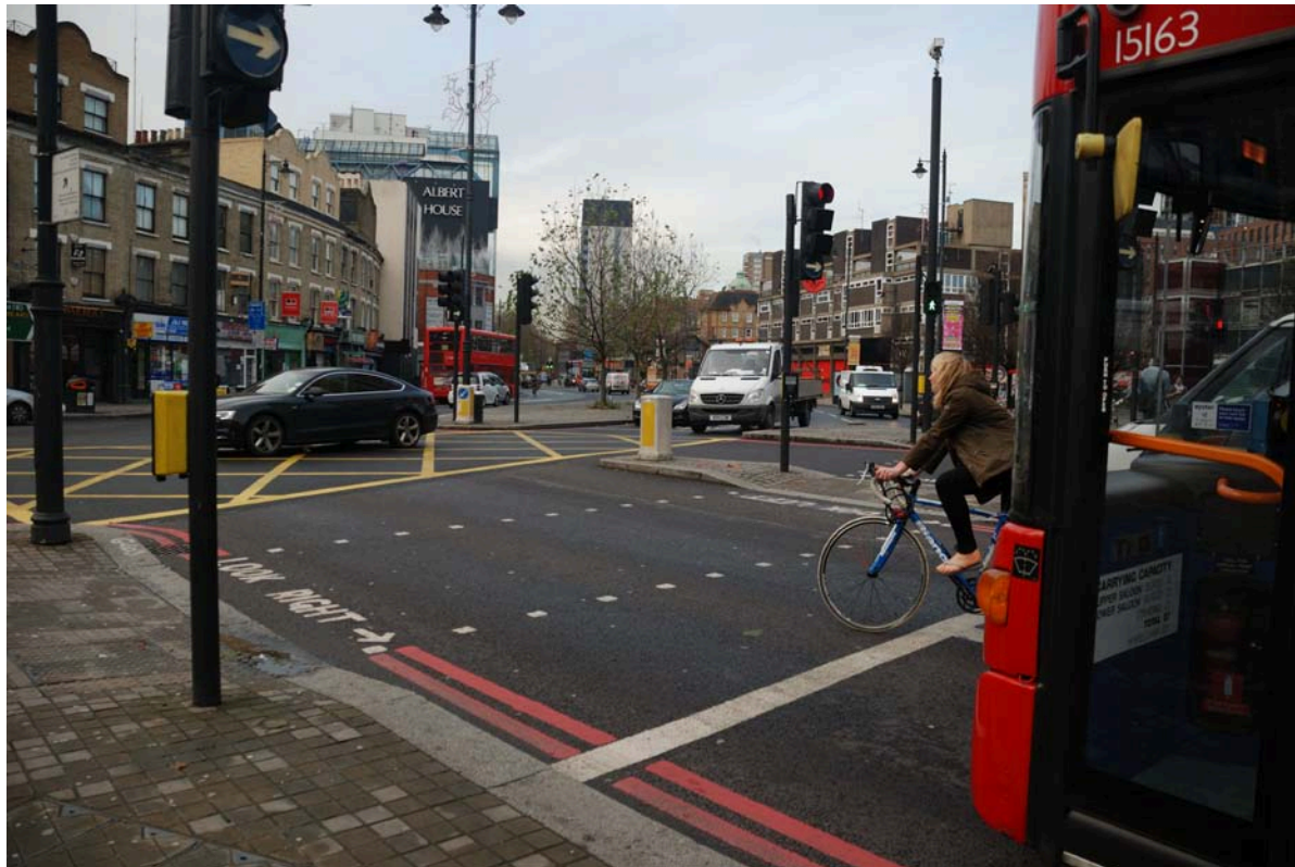
'Apex' junction, Shoreditch - example of a junction that will change
